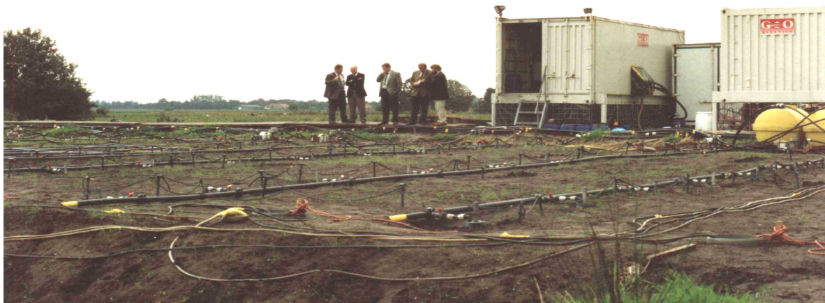
Figure 3. Electro-reclamation of cadmium polluted soil in a temporary lagoon
